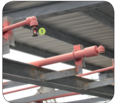
1 Sprinkler system (bulb and nozzle type)
