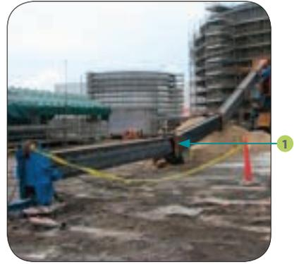
1 Damaged crane boom
