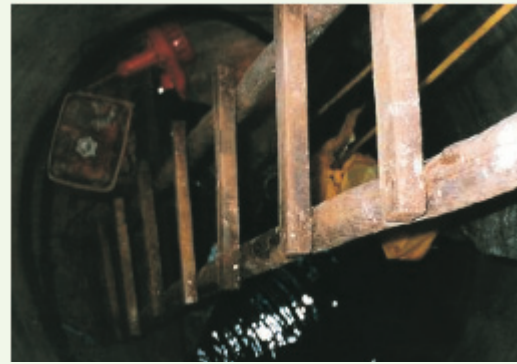
Position of the petrol-driven pump inside the manhole
