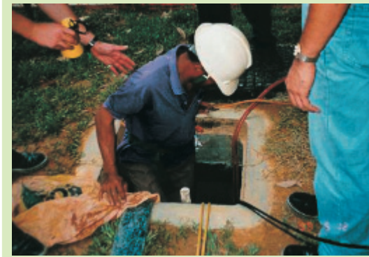
Posed picture showing how the worker entered the manhole
