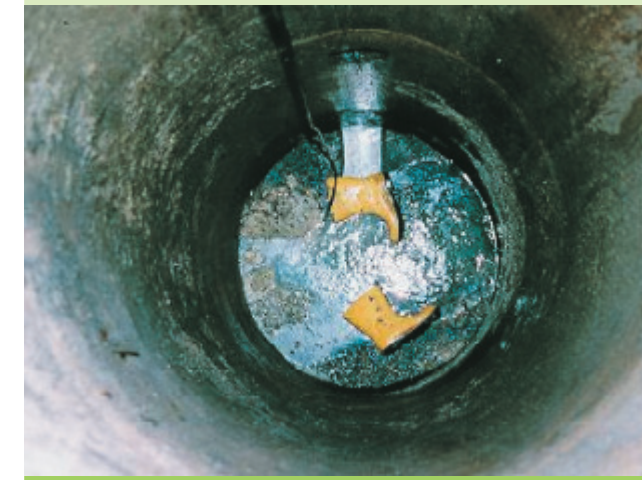
Conditions inside the sewer manhole
